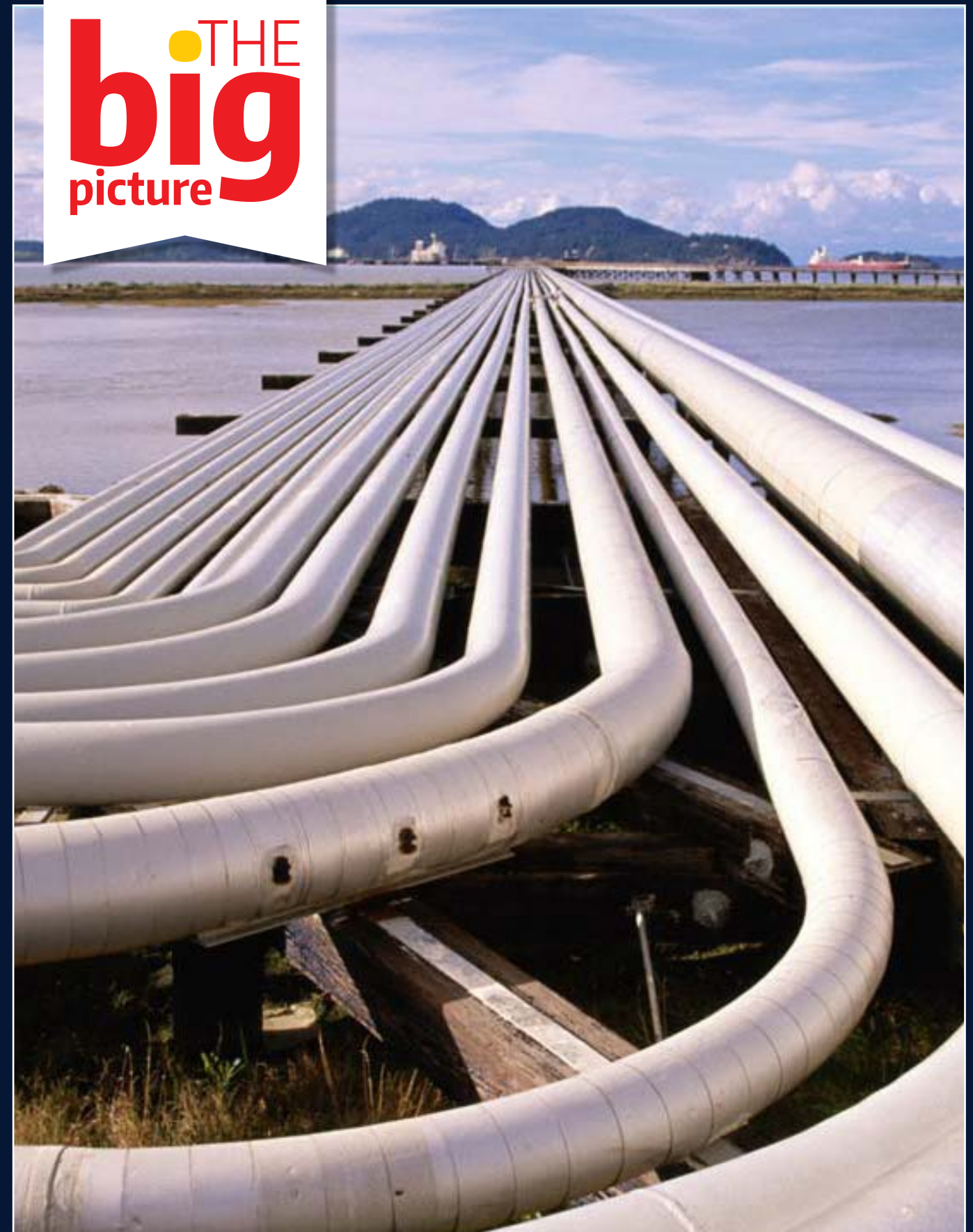
■ Nigeria AKK Pipeline Project
